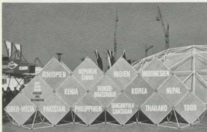
9. The display units inside the tents were composed of "Mero" standard components, forming octahedrons and tetrahedrons. In the foreground, a combination of table and glass pyramids; in the background, a number of larger units.
